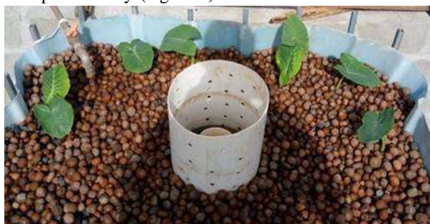
Fig. 8: Filter with stone gravel and expanded clay.
