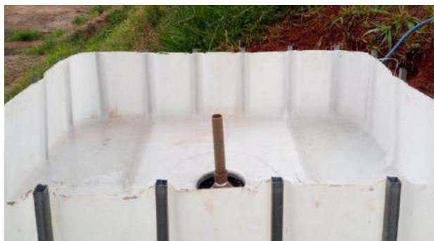
Fig. 7: Rhizospheric filter with water leveler.
