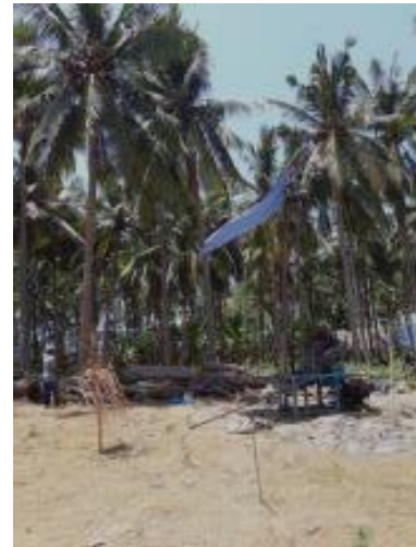
Fig.9: Drilling on Line 3 Point 99.75
