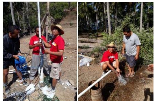
Fig.10: Testing of Pump Installation in Drilling Well
