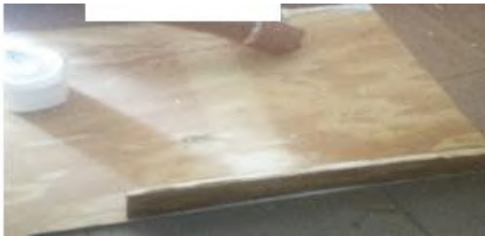
Fig.3: Assembly of plywood
