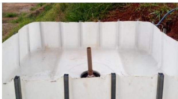
Fig. 7: Rhizospheric filter with water leveler.
